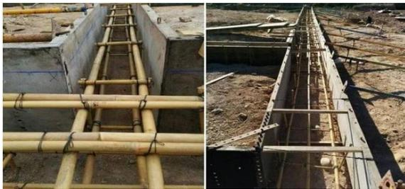
The details on how bamboo is efficient in replacement for steel reinforcement in concrete
